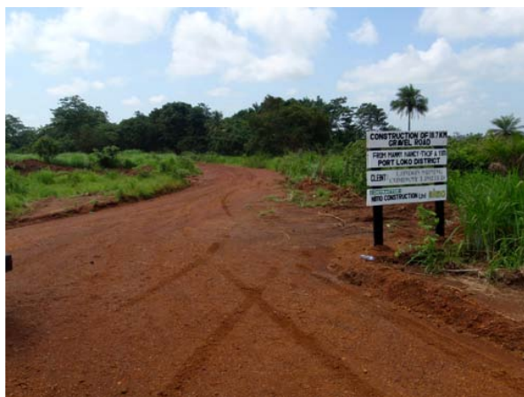
Construction of 18km Marampa haul road
